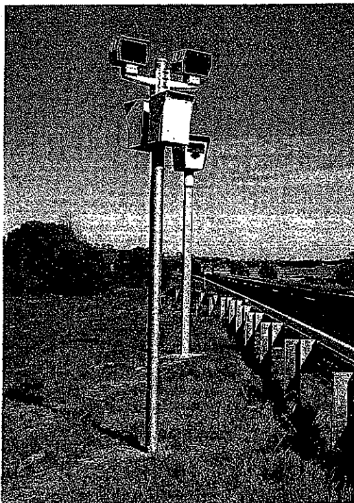
Pole Mounted Point to Point Station with Heavy-Duty High Repetition Rate IR Flash System
