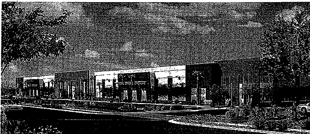
Redflex will soon relocate to this new state-of-the-art facility in Phoenix
